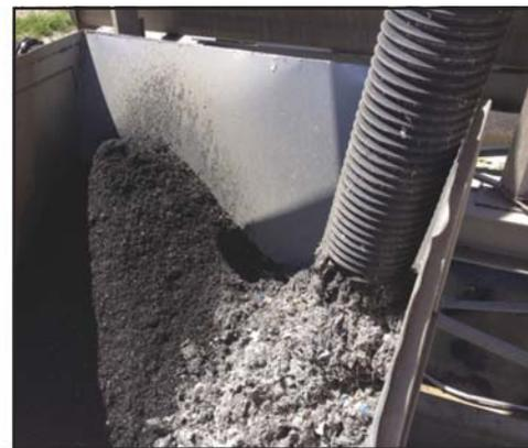
Figure 26. Central District Wastewater Treatment Plant Lakeside Raptor Screens for North District Wastewater Treatment Plant Sludge
